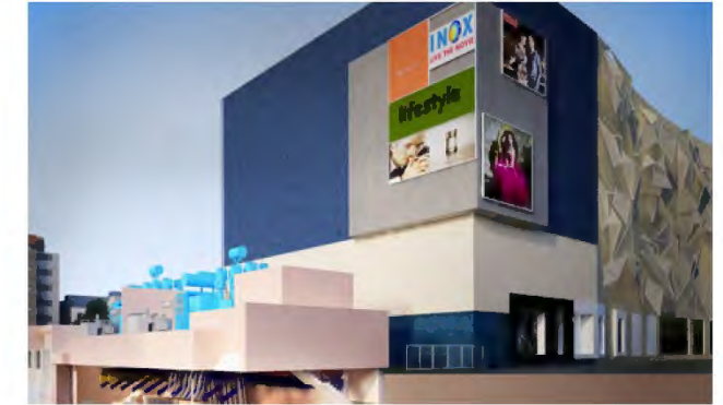
Underground 132 kV SS at 'Quest Mall'
