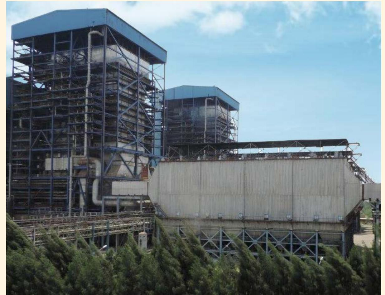
Electrostatic Precipitator used for Reducing Air Emissions
