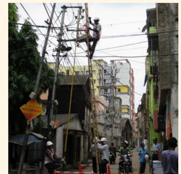
Use of Telescopic Voltage Testing cum Earthing Rod and 6-Way Shorting Clip at Site
